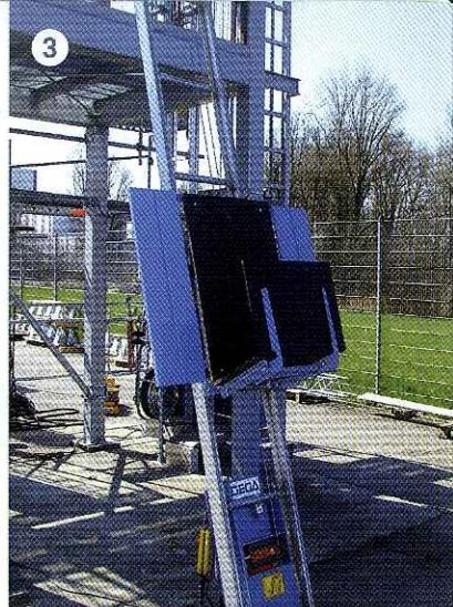
① The solar platform is especially equipped with foam cushioning. The flexibly adjustable fixing grants safe transport.
